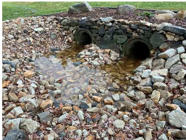
64 Gundalow - 2 (Drainage Course)
