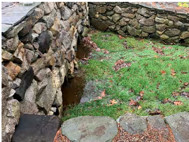
4 Brickyard Circle - 1 (Drainage Course)
