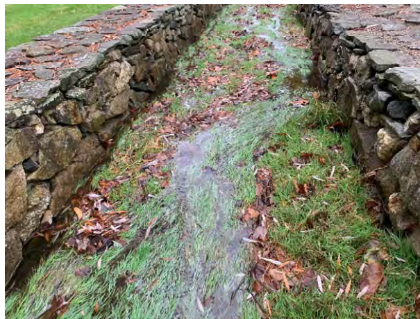
4 Brickyard Circle - 2 (Drainage Course)
