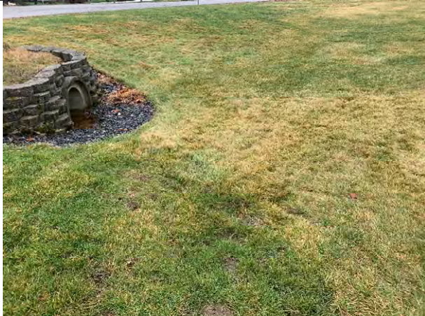
29 Gundalow - 1 (Drainage Area)
