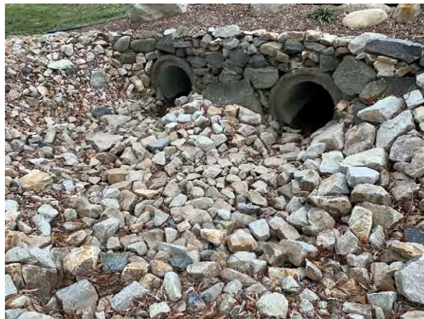
64 Gundalow - 2 (Drainage Course)
