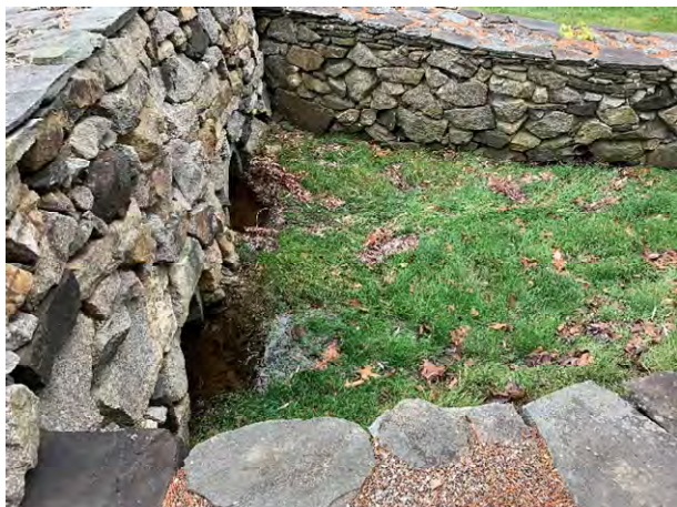
4 Brickyard Circle - 1 (Drainage Course)
