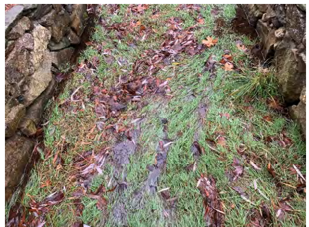
4 Brickyard Circle - 2 (Drainage Course)
