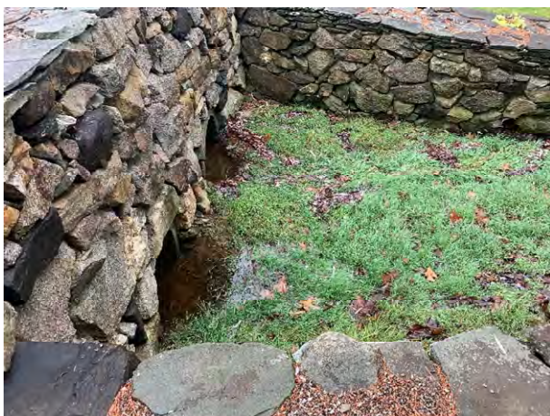
4 Brickyard Circle - 1 (Drainage Course)
