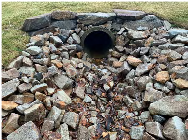
64 Gundalow - 1 (Drainage Course)
