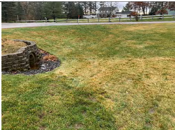
29 Gundalow - 1 (Drainage Area)
