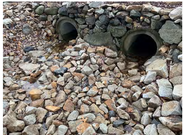
64 Gundalow - 2 (Drainage Course)
