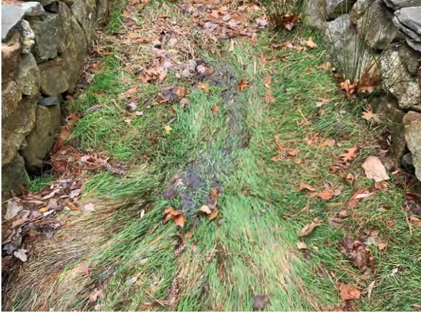
4 Brickyard Circle – 3 (Drainage Course)
