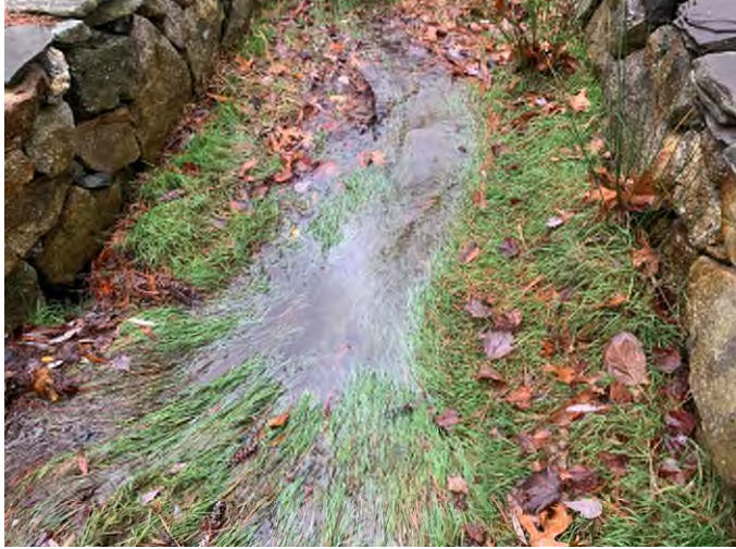
4 Brickyard Circle – 3 (Drainage Course)
