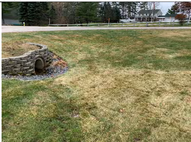
29 Gundalow - 1 (Drainage Area)
