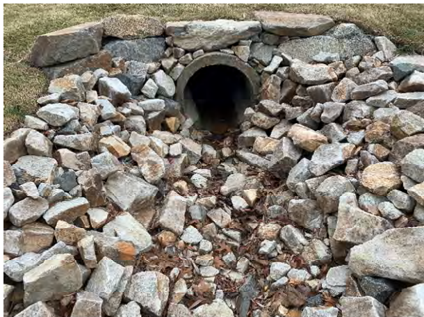
64 Gundalow - 1 (Drainage Course)
