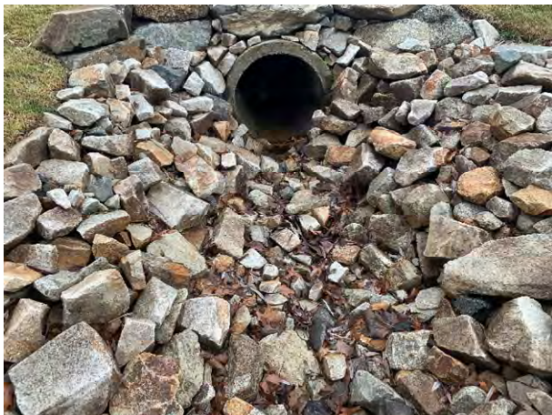
64 Gundalow - 1 (Drainage Course)
